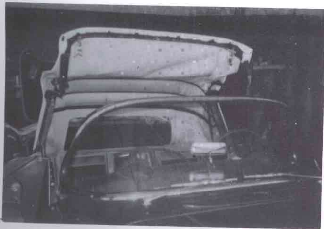
June 1974 — Adjusting for final fit on soft top installation.
