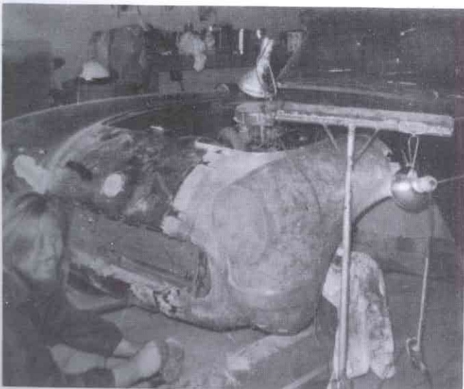
Mickey puts finishing touches to fiberglass repair between head light and grill shell — somehow one of Mickey's music stands got in the set to support the light fixture.
